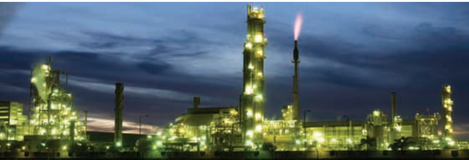
Egyptian Fertilizer Company Ammonia Plant
