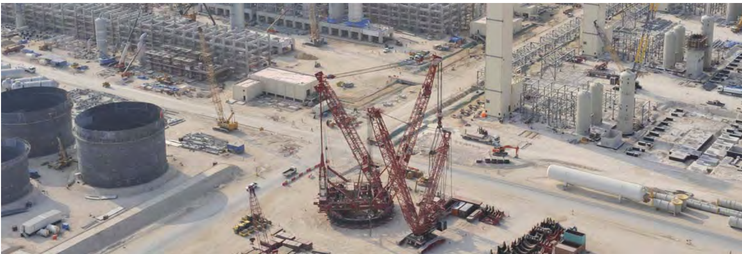
Shell's Pearl GTL plant under construction in Ras Laffan
